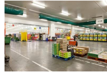
Medium & low Temperature Food Storage (0°C to -21°C) Using secondary glycol solutions
